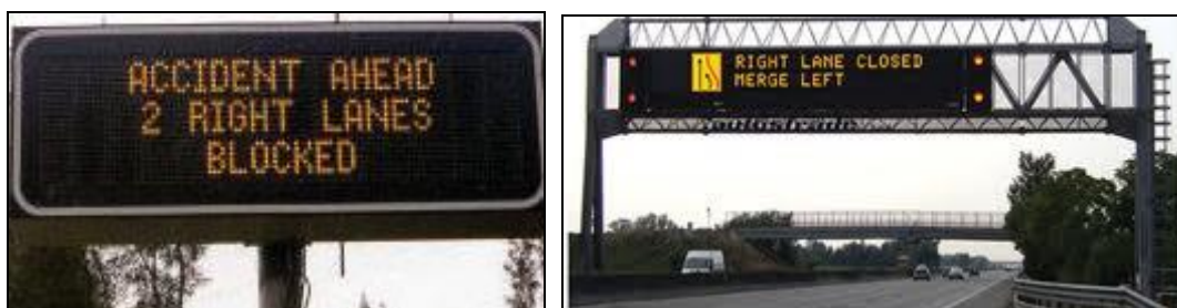
Figure 8-19: Example – Variable Message Sign Boards
