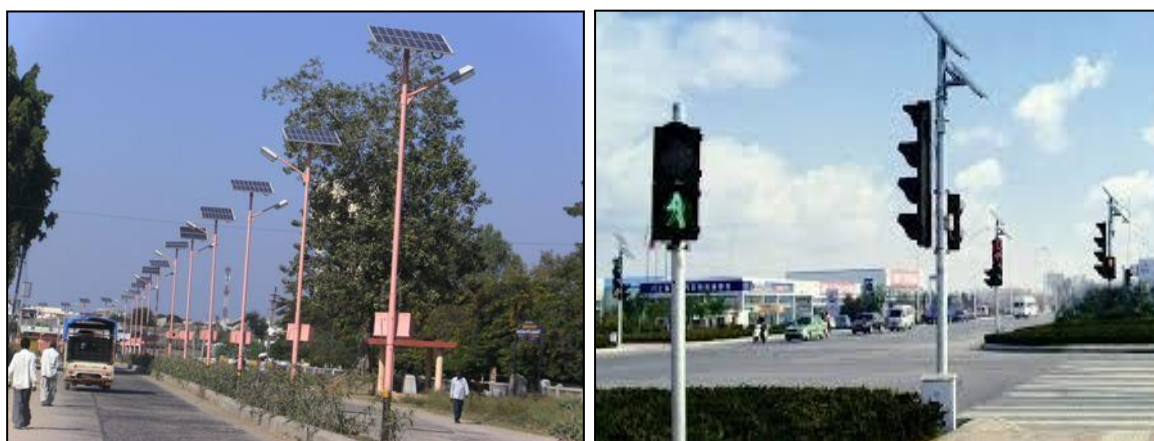
Figure 8-26: Solar Lights and Solar Signals
